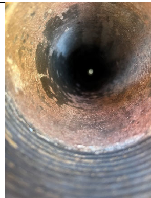
Well 1 - Old carbon steel beginning to oxidize.
