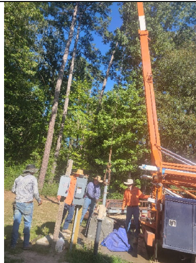
Well 1 - Removing old carbon steel pipe.
