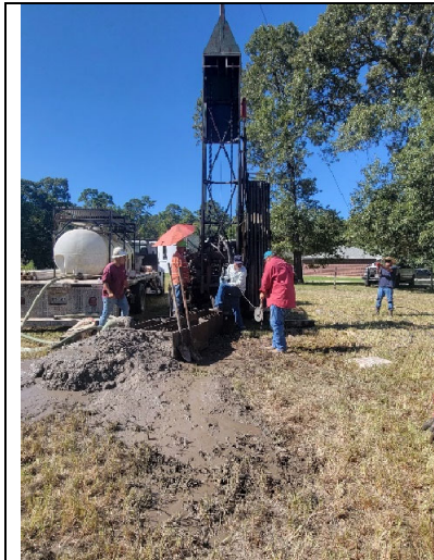
Well 2 – drilling pilot hole.
