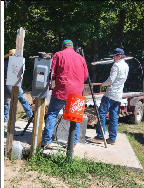
Well 1 – TV Camera about to be inserted into well 1.
