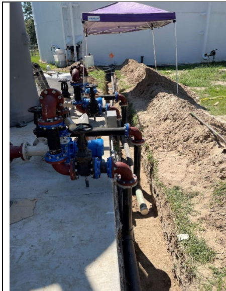
Transfer pump progress.
