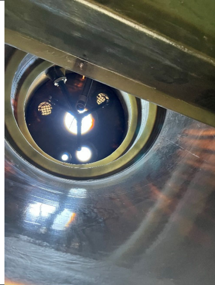
Inside of Filter Tank
