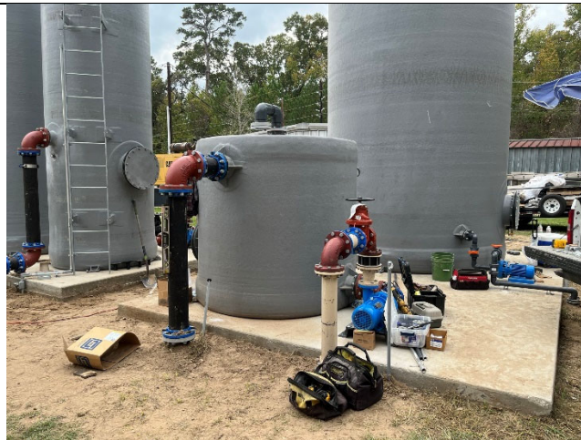
Surge tank piping and surge transfer pump install.
