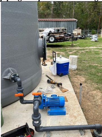
Holding tank piping and transfer pump install.
