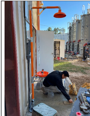
Safety shower install & filter tank piping complete in the background.
